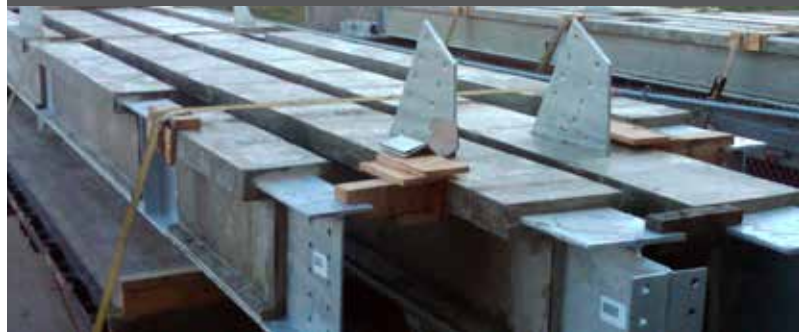
PYROCRETE 241 APPLIED OFFSITE AND TRANSPORTED TO JOBSITE.
