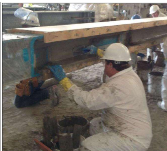
FINISH PYROCRETE WITH USE OF FORM GUIDES
