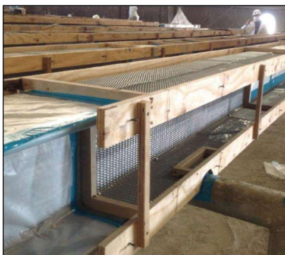
FORMS SET TO REQUIRED THICKNESS
