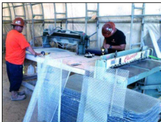
PRE-CUT LATH PRIOR TO APPLICATION
