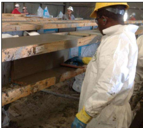
APPLIED PYROCRETE FINISHED WITH A TROWEL
