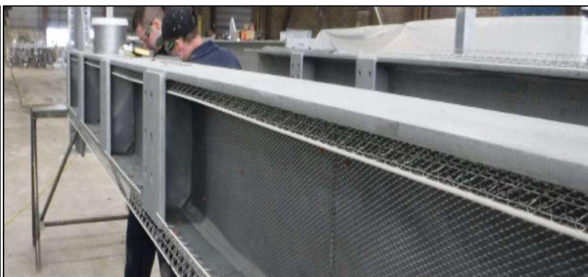
CORNER BEAD INSTALLED FOR THICKNESS CONTROL
