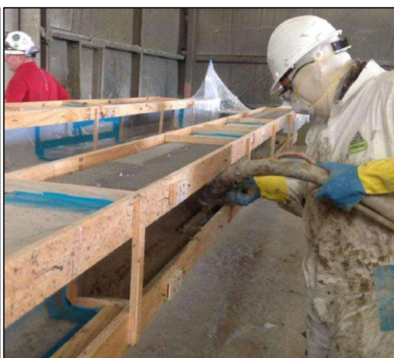
PYROCRETE SPRAY APPLIED TO REQUIRED THICKNESS
