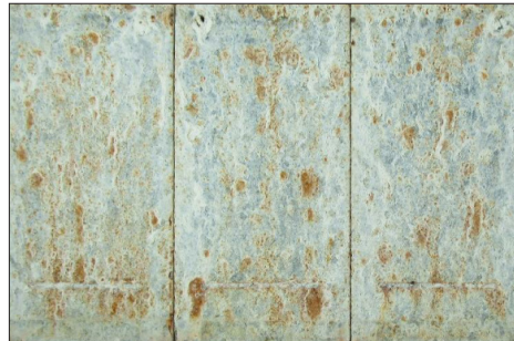
Galvanized panels after 4200 hours ISO 12944-9 CX testing.
