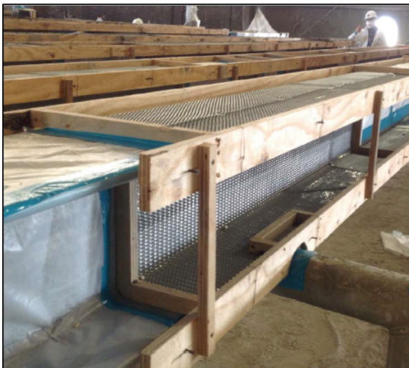
FORMS SET TO REQUIRED THICKNESS
