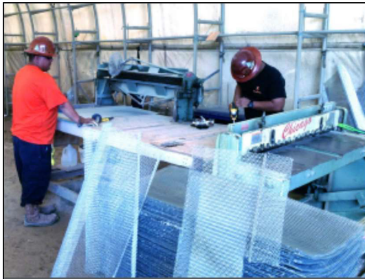
PRE-CUT LATH PRIOR TO APPLICATION
