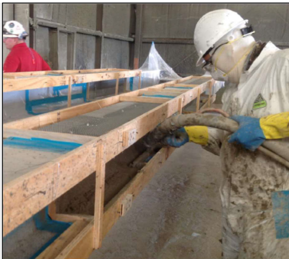
PYROCRETE SPRAY APPLIED TO REQUIRED THICKNESS
