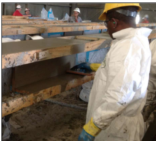
APPLIED PYROCRETE FINISHED WITH A TROWEL
