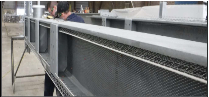
CORNER BEAD INSTALLED FOR THICKNESS CONTROL
