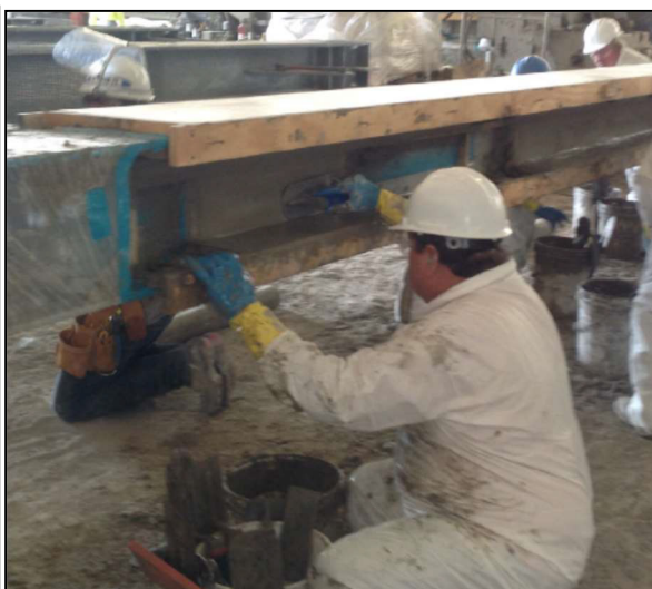
FINISH PYROCRETE WITH USE OF FORM GUIDES
