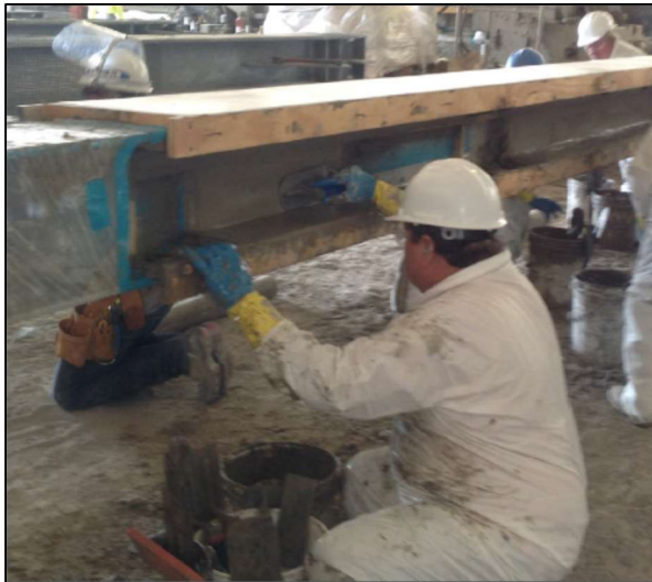
FINISH PYROCRETE WITH USE OF FORM GUIDES
