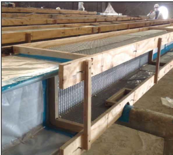
FORMS SET TO REQUIRED THICKNESS
