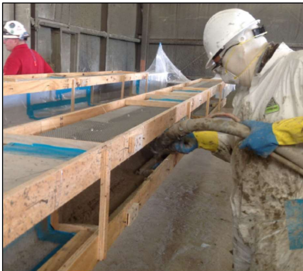
PYROCRETE SPRAY APPLIED TO REQUIRED THICKNESS
