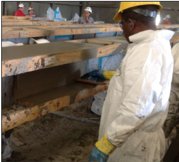
APPLIED PYROCRETE FINISHED WITH A TROWEL
